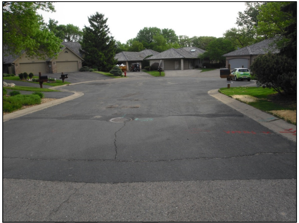
Photo 2: Existing Pavement Condition
