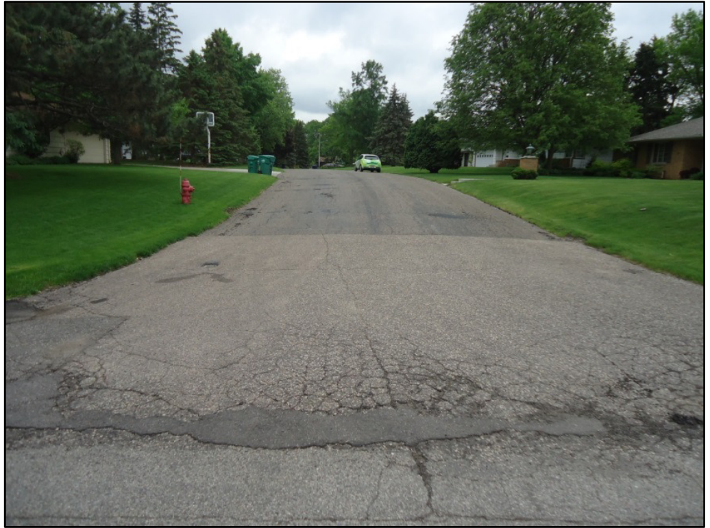
Photo 2: Existing Pavement Condition
