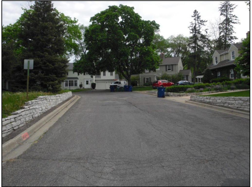
Photo 2: Existing Pavement Condition
