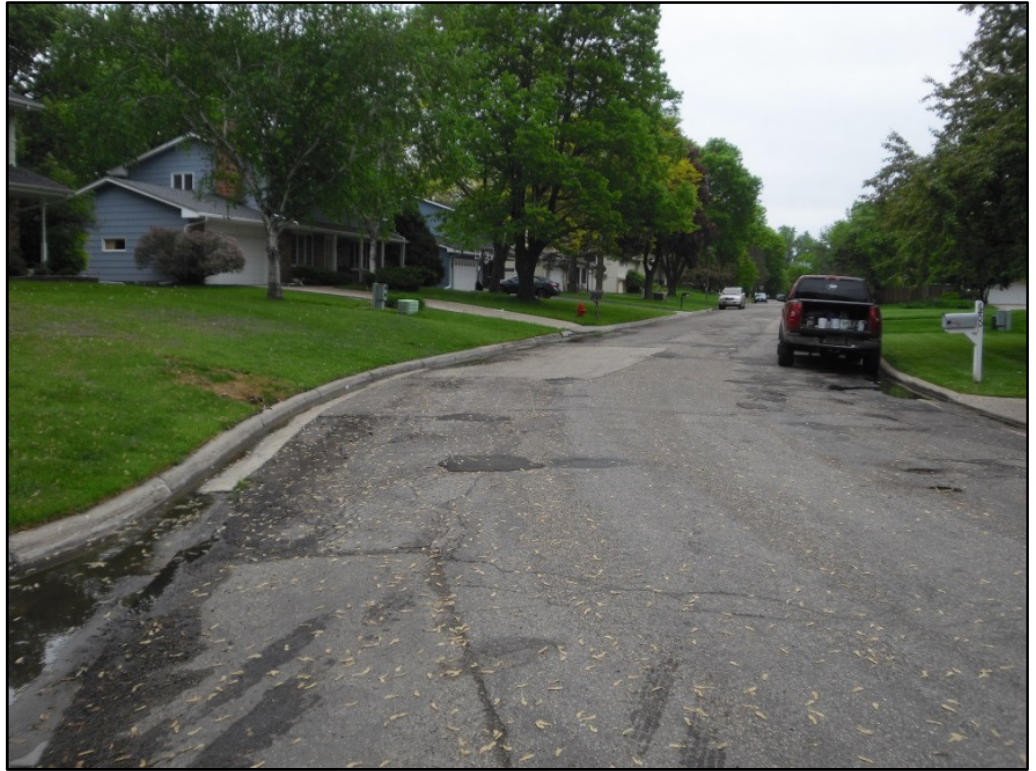
Photo 2: Existing Pavement Condition
