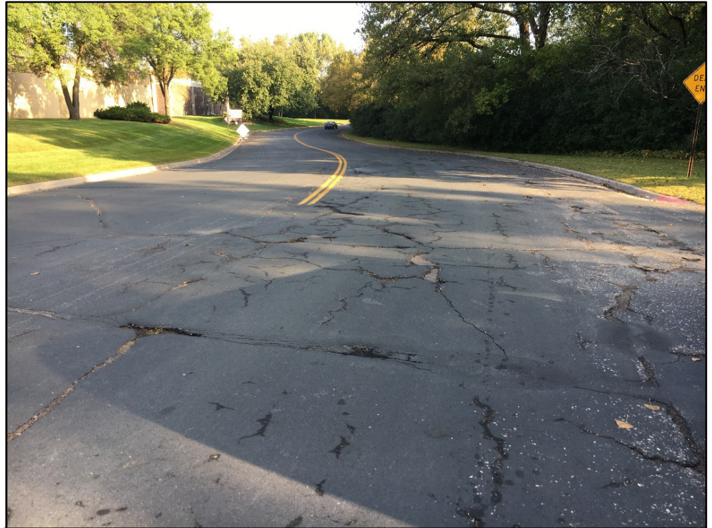
Photo 2: Existing Pavement Condition
