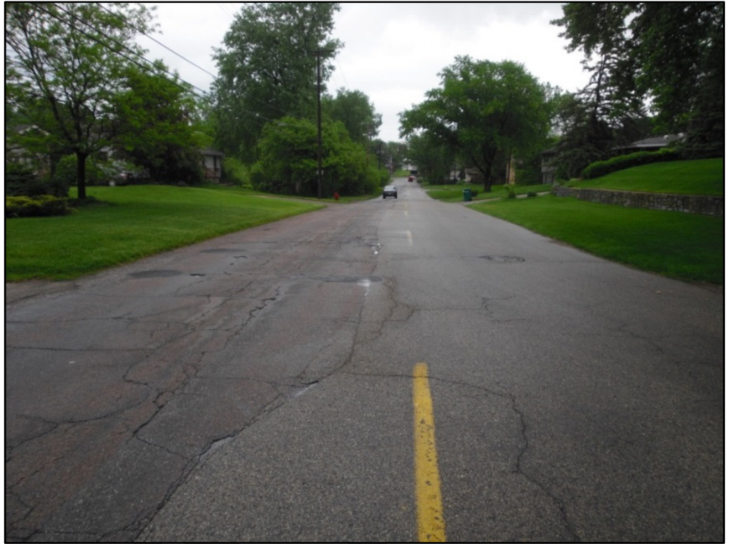
Photo 2: Existing Pavement Condition
