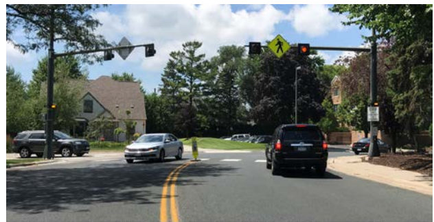
Photo: Overhead flashing lights with RRFB at W 51 st St and Halifax Ave
