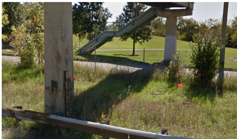
Figure 4: Existing Column Damage
