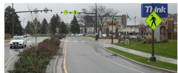
Photo: Pedestrian crosswalk which includes amber flashers on pedestrian sign to the right and above the crosswalk.
