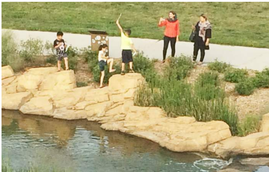
The design of this stormwater collection and treatment facility in Lincoln, Nebraska, provides beauty and landscape for public enjoyment.
