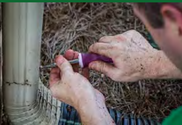
Redirecting gutter downspouts towards vegetated areas
