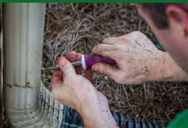
Redirecting gutter downspouts towards vegetated areas
