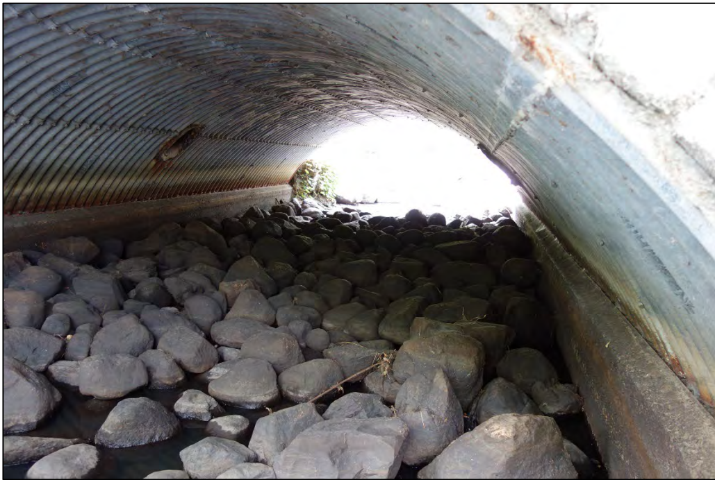
Detail of the east limestone headwall and metal arch, looking southwest (top). Looking west beneath the bridge. Circular areas where a pipe once penetrated the arch are visible in the background. Both photographs are from 2021.
