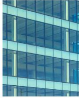
HYBRID WINDOW WALL - SSG SYSTEM
