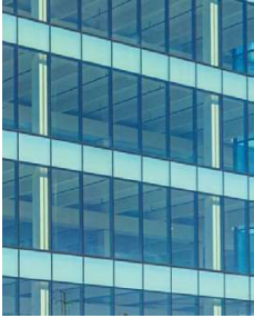
HYBRID WINDOW WALL - SSG SYSTEM
