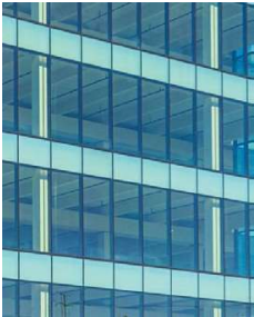
HYBRID WINDOW WALL - SSG SYSTEM
