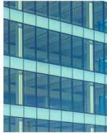
HYBRID WINDOW WALL - SSG SYSTEM
