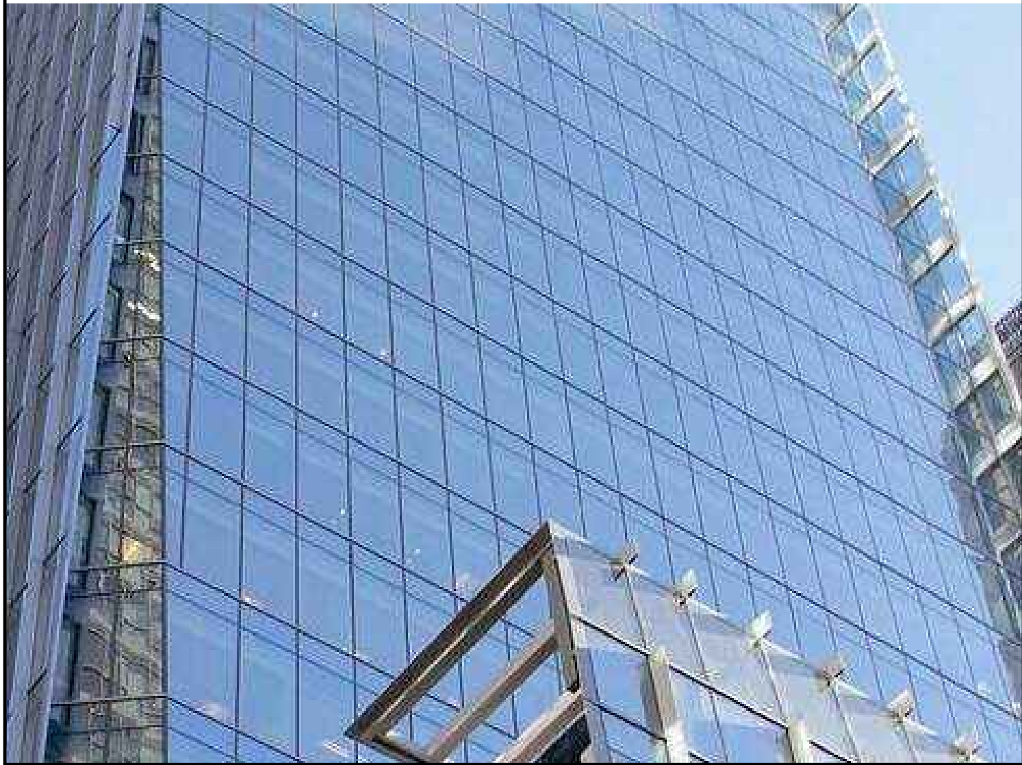
EXTERIOR GLASS ENCLOSURE HYBRID WINDOW WALL - SSG SYSTEM
