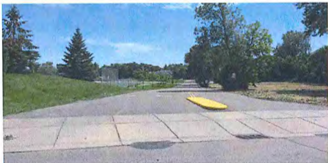
Figure 3.49 Existing northern entrance/exit to OLG off of Eden Avenue, showing a completely uncontrolled intersection condition and oversized vehicular facilities for average traffic needs.
