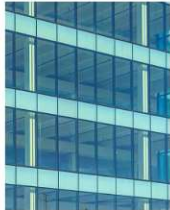
HYBRID WINDOW WALL - SSG SYSTEM
