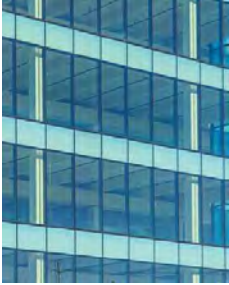
HYBRID WINDOW WALL - SSG SYSTEM
