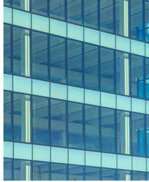
HYBRID WINDOW WALL - SSG SYSTEM
