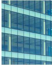
HYBRID WINDOW WALL - SSG SYSTEM
