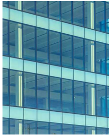
HYBRID WINDOW WALL - SSG SYSTEM
