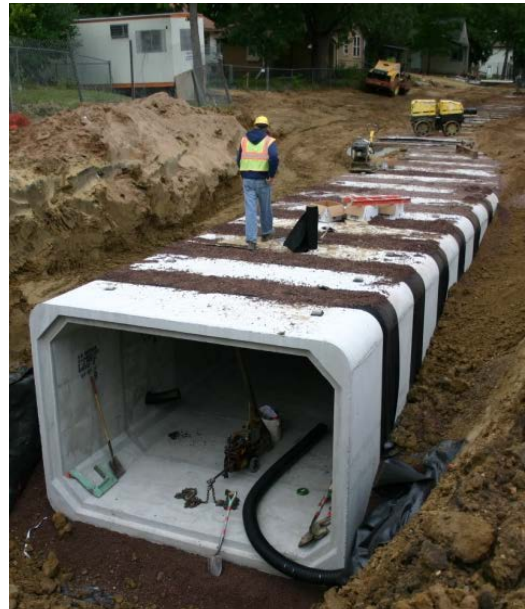
Figure 2 Example of an underground storage vault (37 th Avenue Greenway, Minneapolis).
