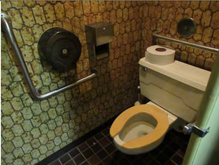
Photo 13: Restroom does not comply with current ADA requirements
