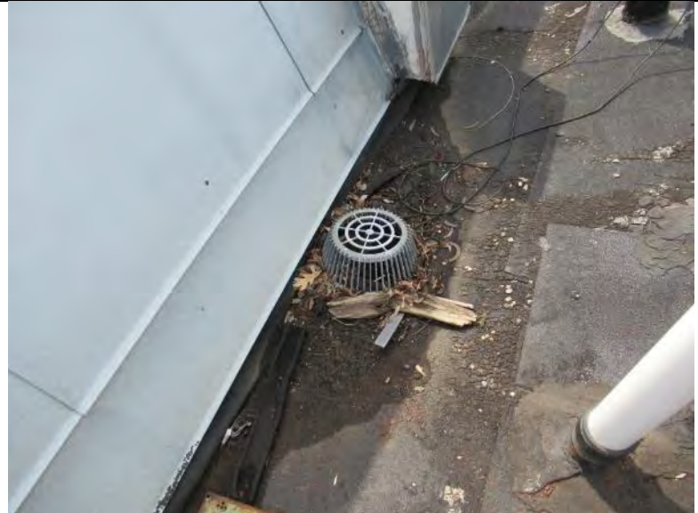
Photo 20: Roof drains only. No overflow roof drains.
