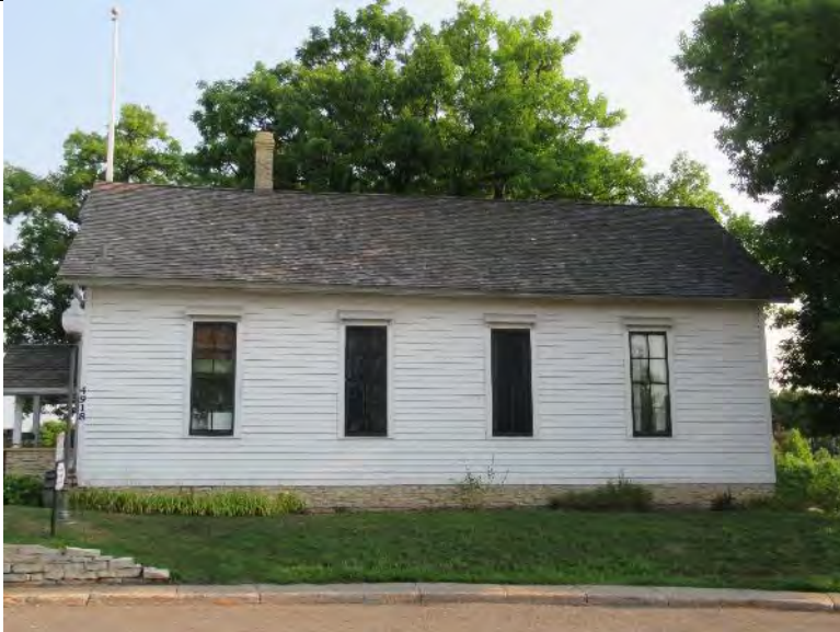
Photo 39: Minnehaha Grange Hall south wall showing lap siding, single-glazed double-hung windows and cedar shingles
