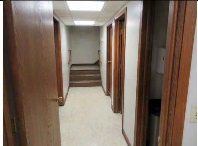
Photo 50: Minnehaha Grange Hall stair tread depth, riser height, and handrails do not comply with current code requirements
