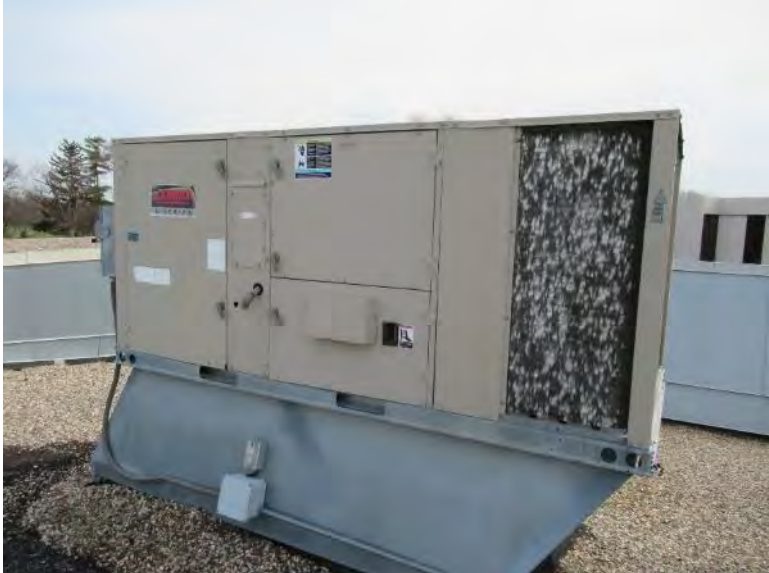
Photo 23: Rooftop equipment requires regular replacement of filters. Vertical ladder roof access does not meet current codes
