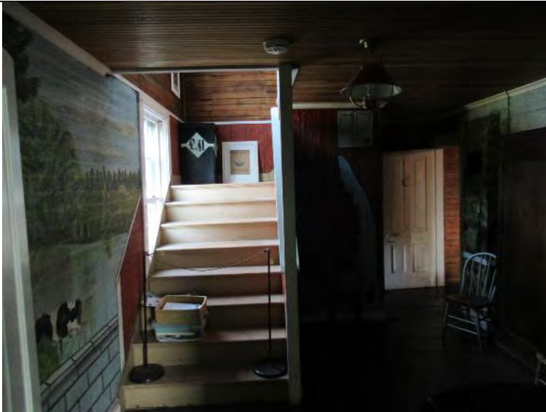
Photo 49: Minnehaha Grange Hall stair tread depth, riser height, and handrails do not comply with current code requirements
