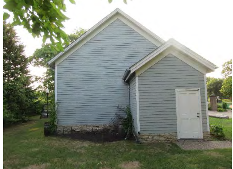
Photo 28: Historic Cahill School west wall showing lap siding and cedar shingles
