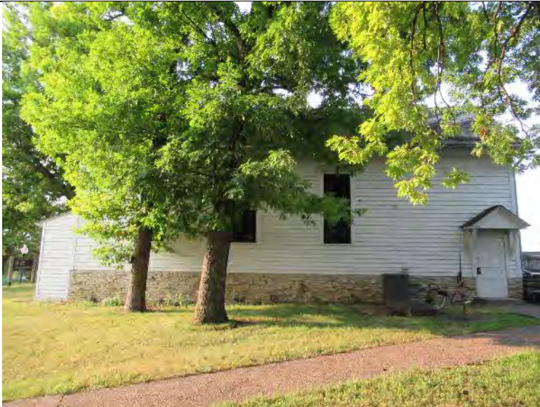
Photo 41: Minnehaha Grange Hall north wall showing lap siding, single-glazed double-hung windows and cedar shingles
