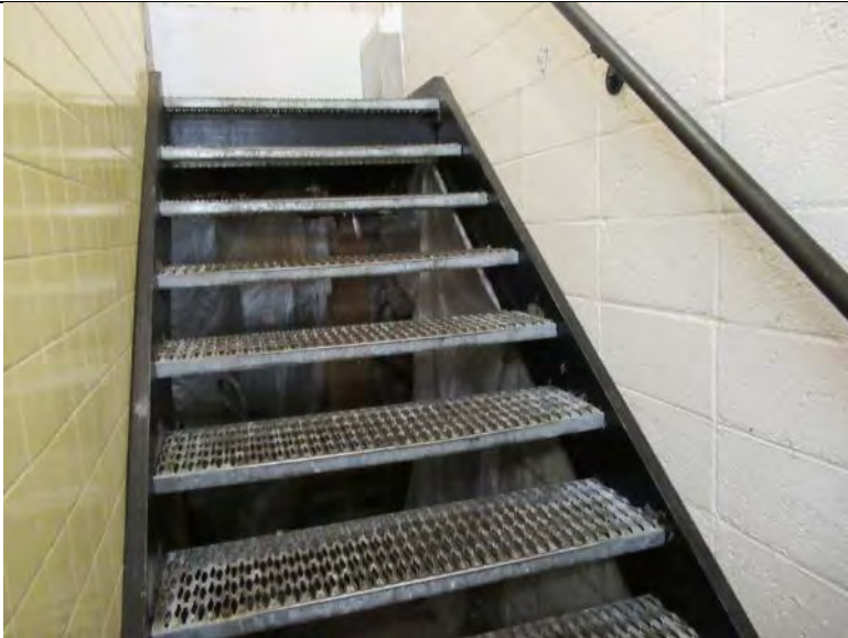
Photo 17: Stair tread depth, riser height, and handrails do not comply with current code requirements
