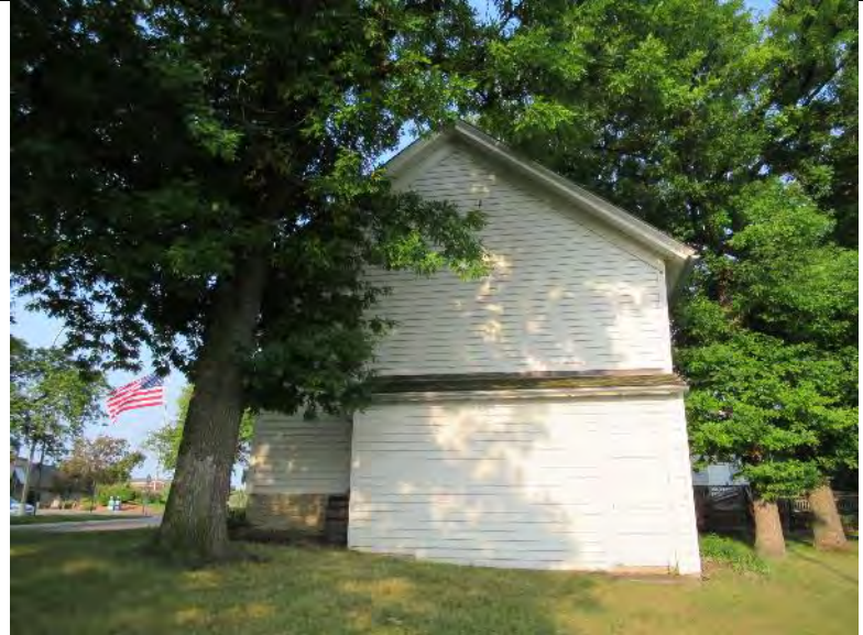
Photo 40: Minnehaha Grange Hall east wall showing lap siding and cedar shingles
