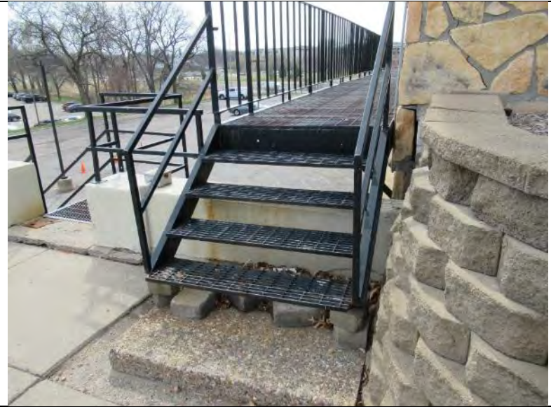
Photo 26: Emergency exit stair tread depth, riser height, and handrails do not comply with current code requirements
