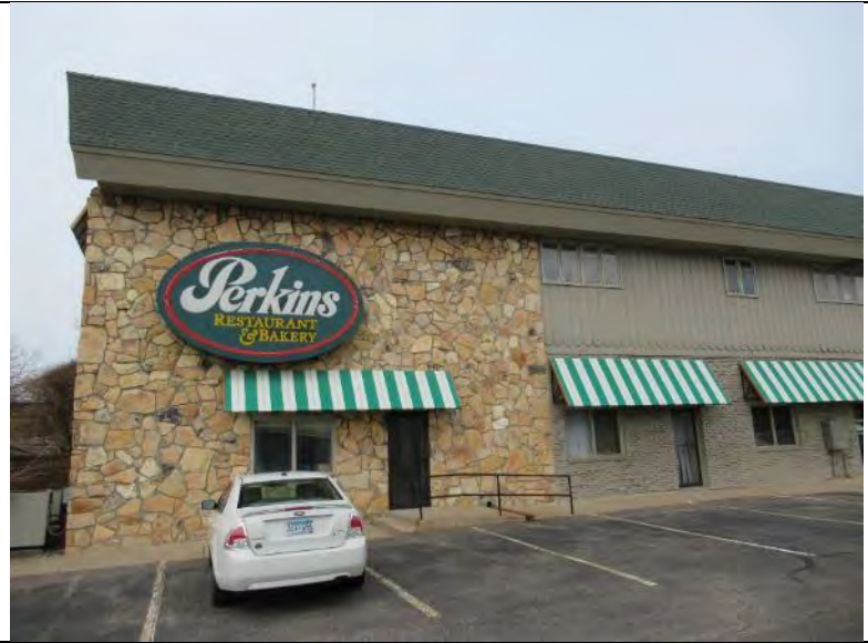
Photo 6: South exterior wall showing stone, brick, wood siding, and shingled mansard roof
