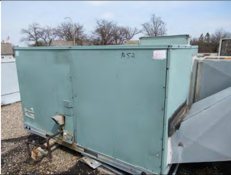
Photo 25: Rooftop equipment requires regular replacement of filters. Vertical ladder roof access does not meet current codes
