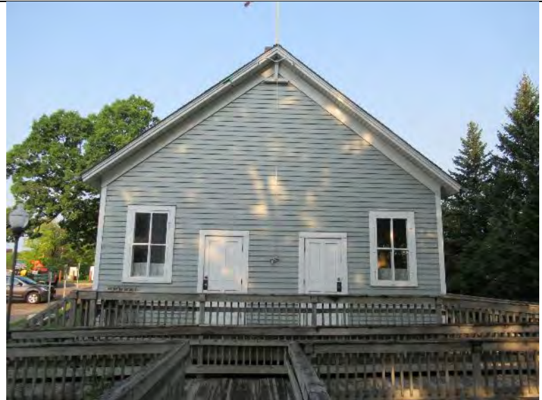
Photo 30: Historic Cahill School east wall showing lap siding, single-glazed double-hung windows and cedar shingles
