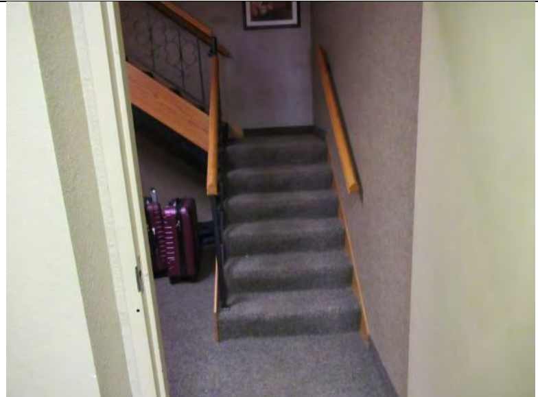
Photo 18: Stair tread depth, riser height, and handrails do not comply with current code requirements
