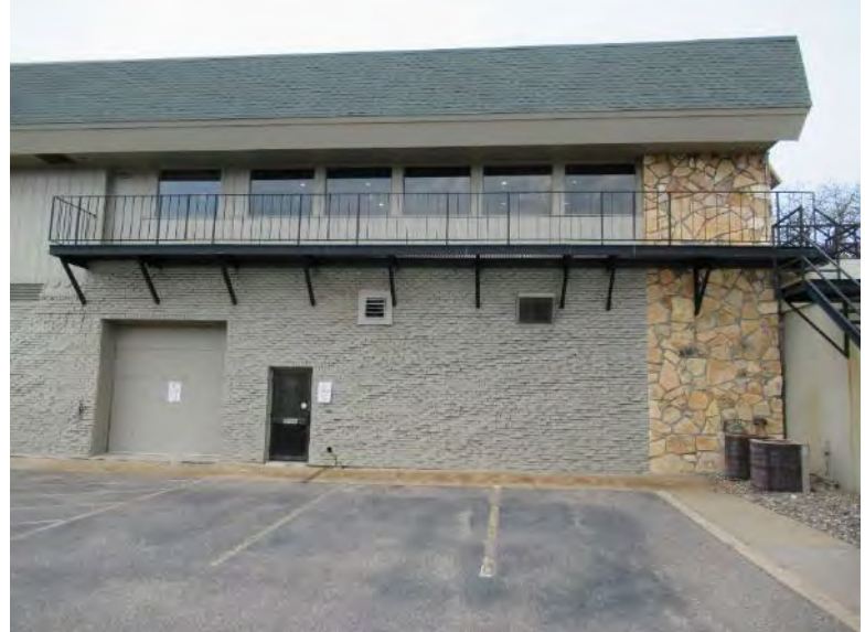
Photo 8: South exterior wall showing stone, brick, wood siding, shingled mansard roof, and emergency exit catwalk
