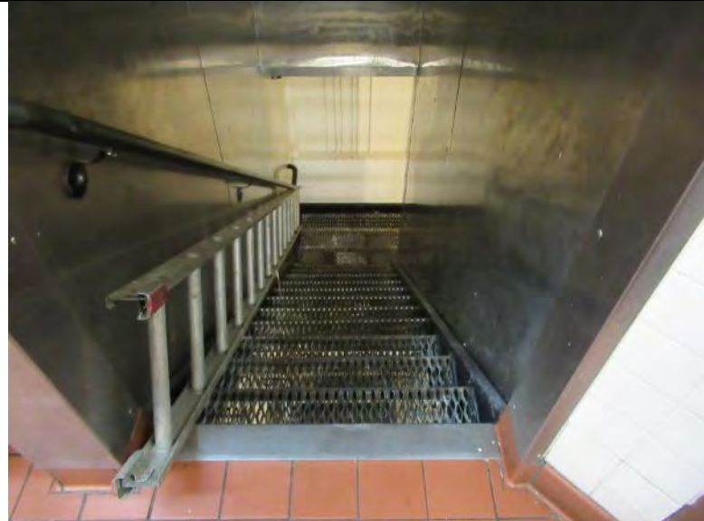
Photo 16: Stair tread depth, riser height, and handrails do not comply with current code requirements
