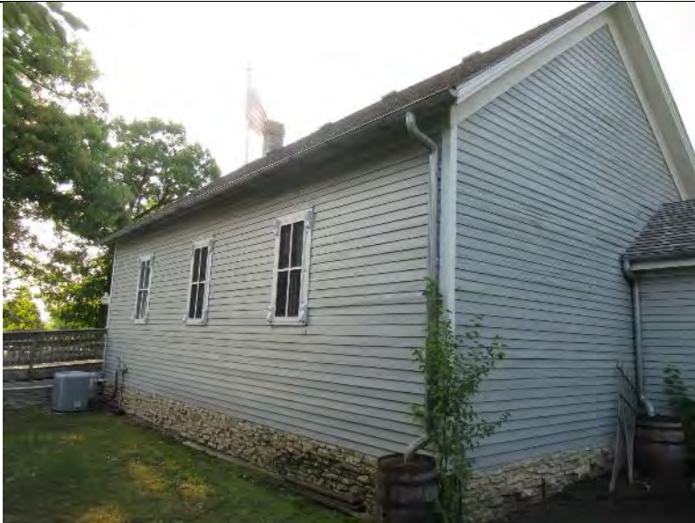
Photo 29: Historic Cahill School north wall showing lap siding, single-glazed double-hung windows and cedar shingles
