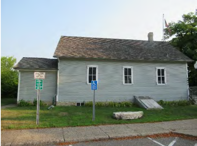
Photo 27: Historic Cahill School south wall showing lap siding, single-glazed double-hung windows and cedar shingles
