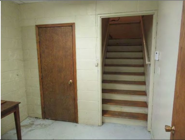
Photo 37: Historic Cahill School stair tread depth, riser height, and handrails do not comply with current code requirements
