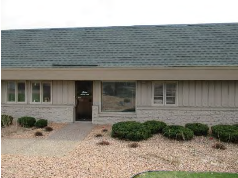
Photo 3: North exterior wall showing brick, wood board and battens, and shingled mansard roof
