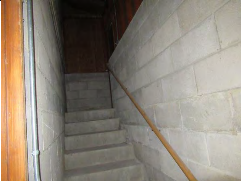
Photo 55: Minnehaha Grange Hall stair tread depth, riser height, and handrails do not comply with current code requirements
