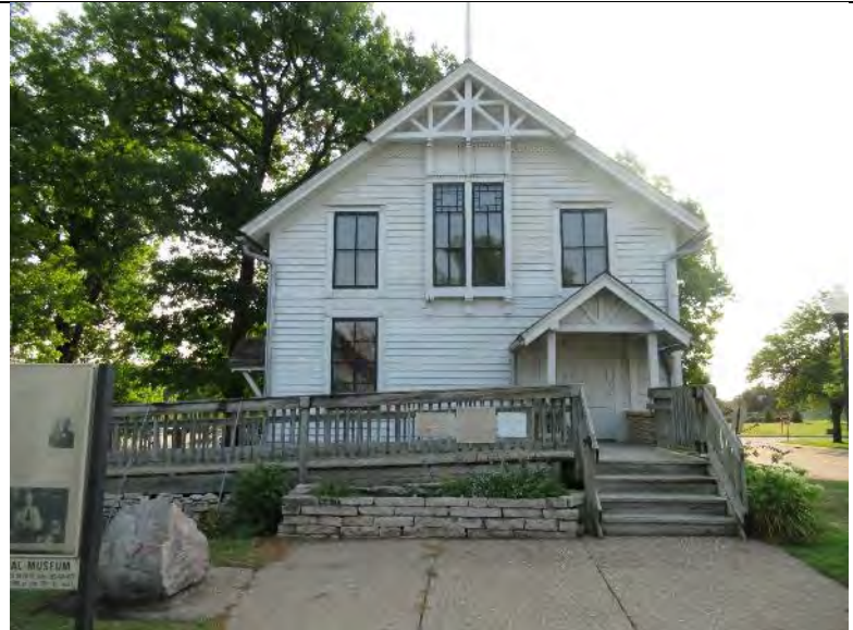
Photo 42: Minnehaha Grange Hall west wall showing lap siding, single-glazed double-hung windows and cedar shingles
