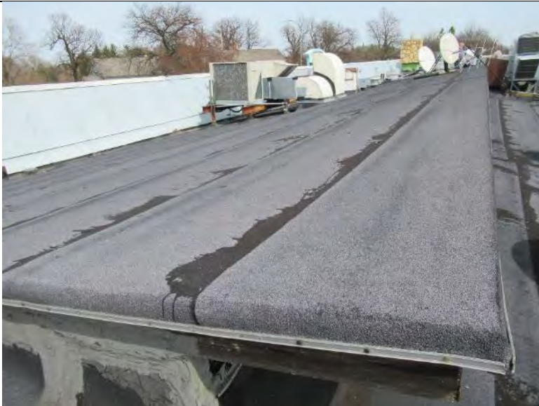
Photo 21: Existing built-up roofing system does not comply with current energy code requirements
