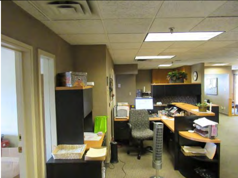
Photo 19: Lighting does not comply with current energy code requirements
