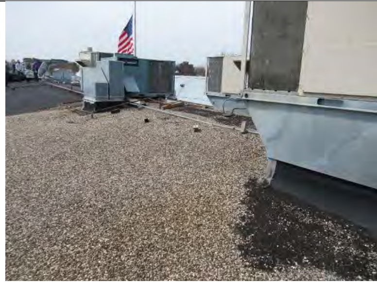
Photo 22: Existing built-up roofing system does not comply with current energy code requirements
