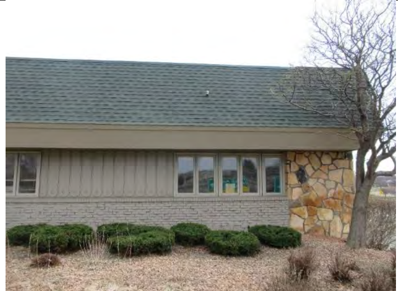
Photo 4: North exterior wall showing brick, stone, wood board and battens, and shingled mansard roof
