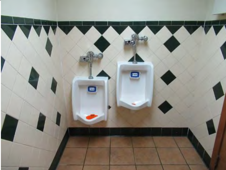
Photo 11: Lower urinal does not comply with ADA clear width requirements
