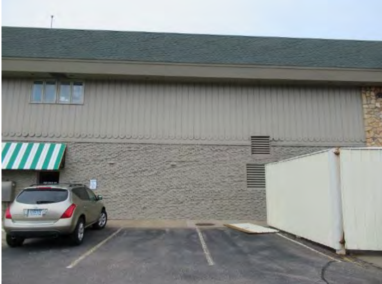
Photo 7: South exterior wall showing stone, brick, wood siding, and shingled mansard roof
