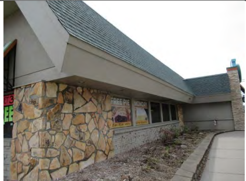
Photo 2: East and north exterior walls showing brick, stone, stucco, and shingled mansards
