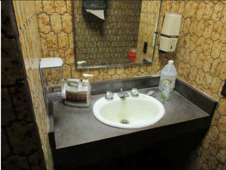
Photo 15: Bottom of mirror is too high and does not comply with current ADA requirements
