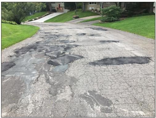
**Photo 2: Existing Bituminous Pavement Condition**
