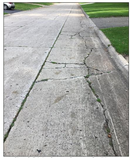
**Photo 3: Existing Concrete Pavement Condition**
