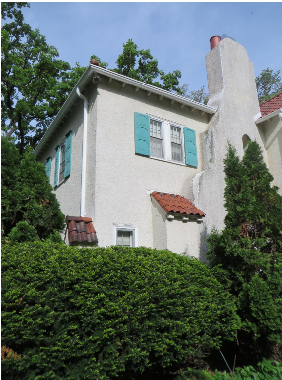
Image 5: Patching of existing stucco does not match color or texture of original stucco, windows and shutters are in need to repair and paint
