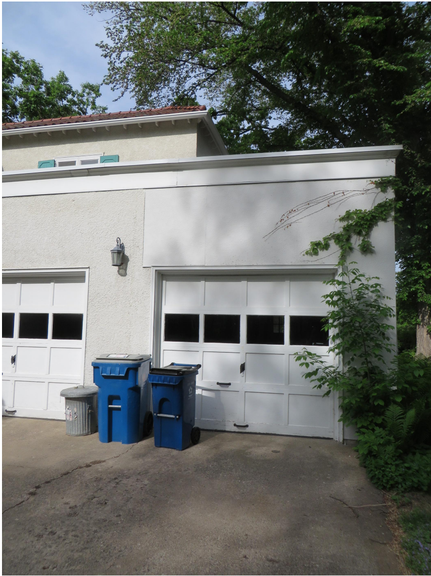
Image 3: 1950s garage addition uses panelized stucco that does not match original stucco
