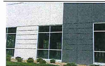
AGGREGATE FINISH EXAMPLE
