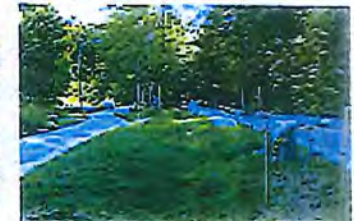
STORMWATER SWALE BETWEEN PATHS
