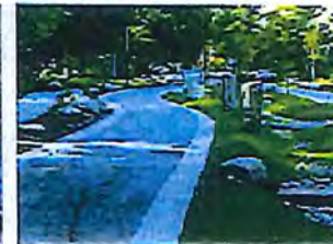
STORMWATER SWALE ADJACENT TO PATH
