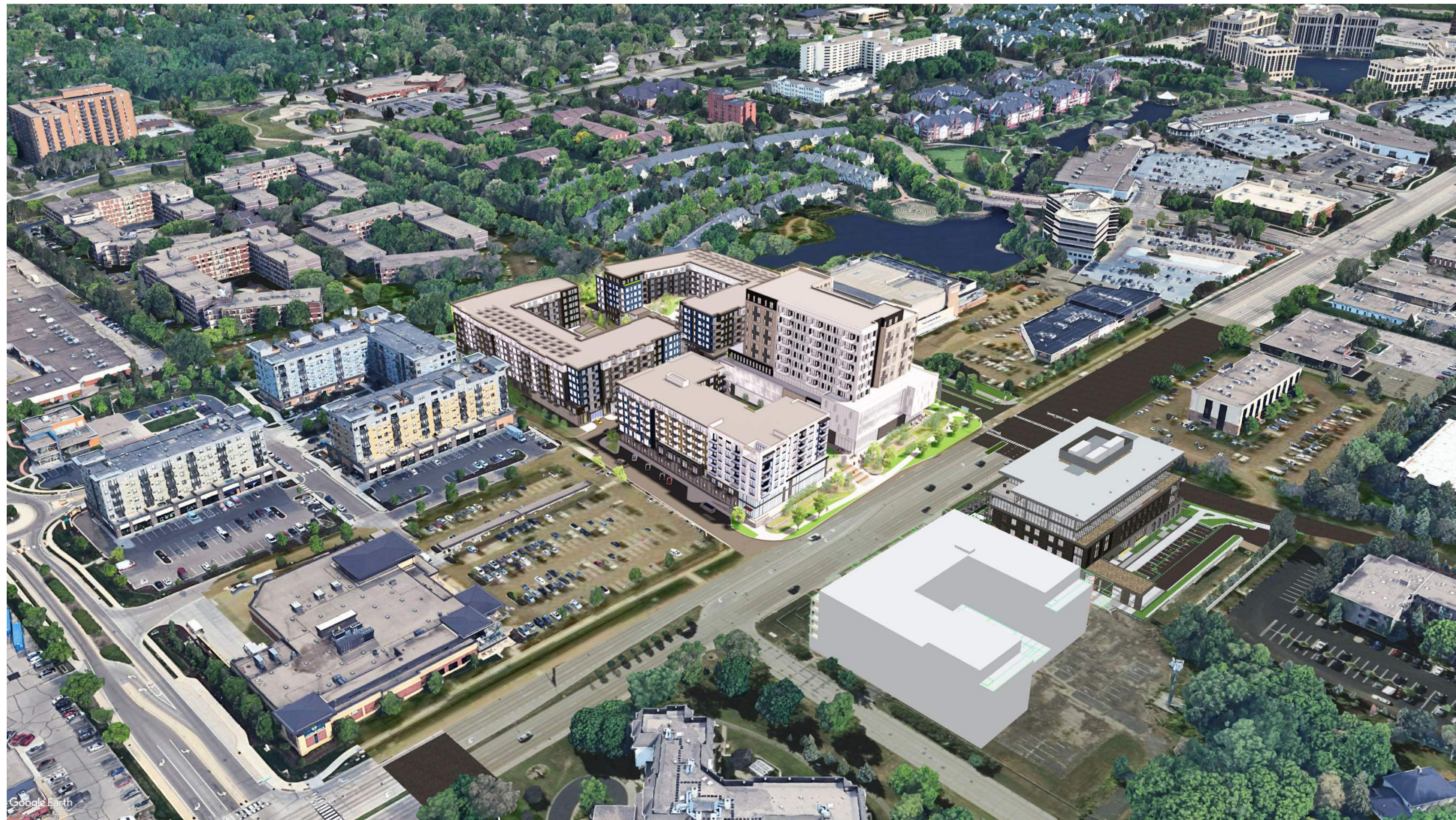
AERIAL - NW CORNER
