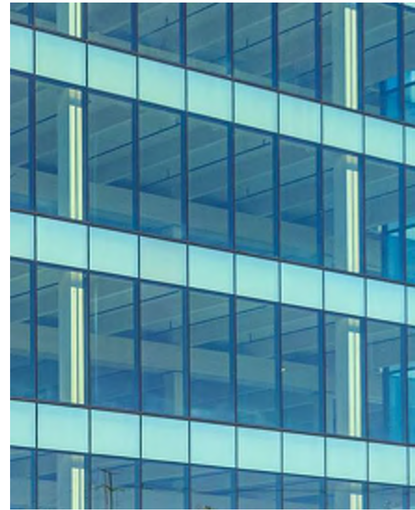
HYBRID WINDOW WALL - SSG SYSTEM (KEYNOTE 8)
