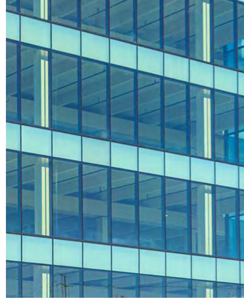
HYBRID WINDOW WALL - SSG SYSTEM
