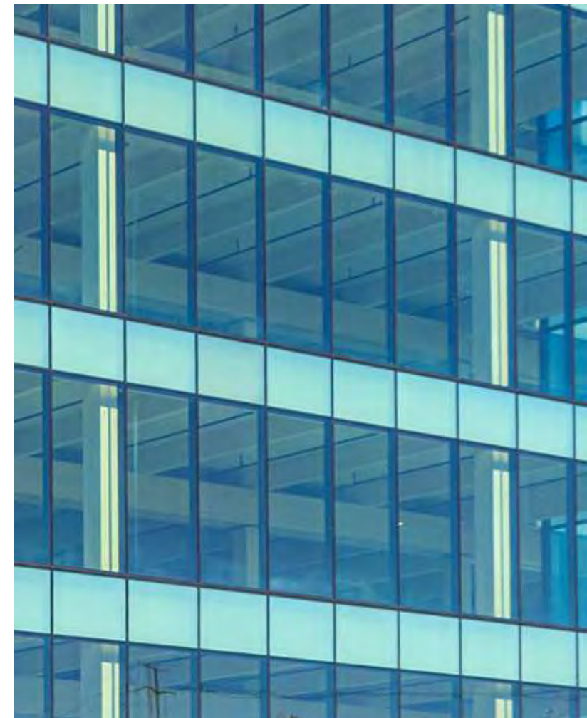
HYBRID WINDOW WALL - SSG SYSTEM
