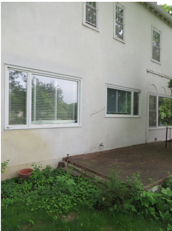
Image 6: Surface cracking seen throughout the existing stucco
