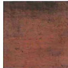
I - Steel Siding
